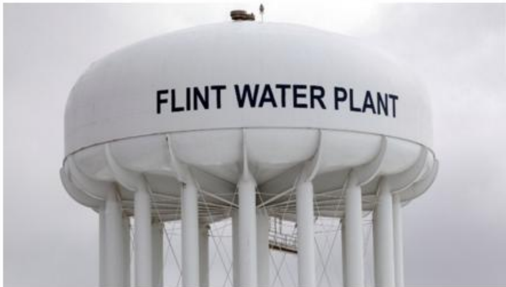
The Flint Water Plant tower.
