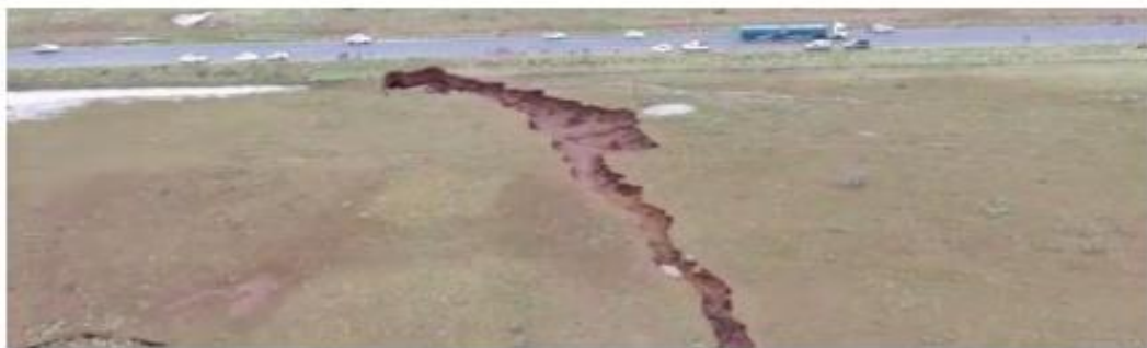
Fissure in Northern Cape, South Africa
