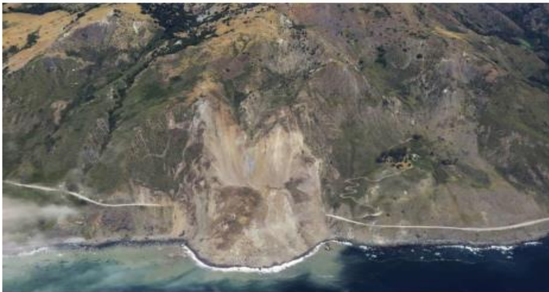
A massive new landslide along California's iconic coastal Highway 1 has buried the road under a 40-foot layer of rock and
