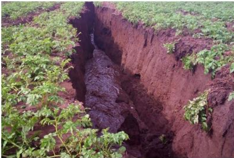
A new giant crack opened up at Moi Ndabi area on the outskirts of Naivasha town. via Nation
