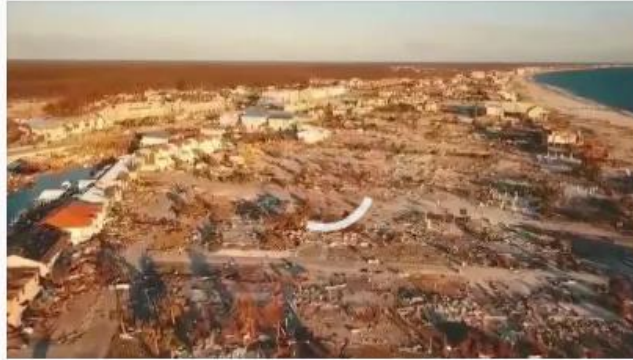
Drone aerial video from Mexico Beach, Florida shows a stretch of the town with almost every structure no longer standing. There was just one confirmed death so far in Mexico Beach, which Hurricane Michael nearly wiped off the map. (Oct. 16) AP
