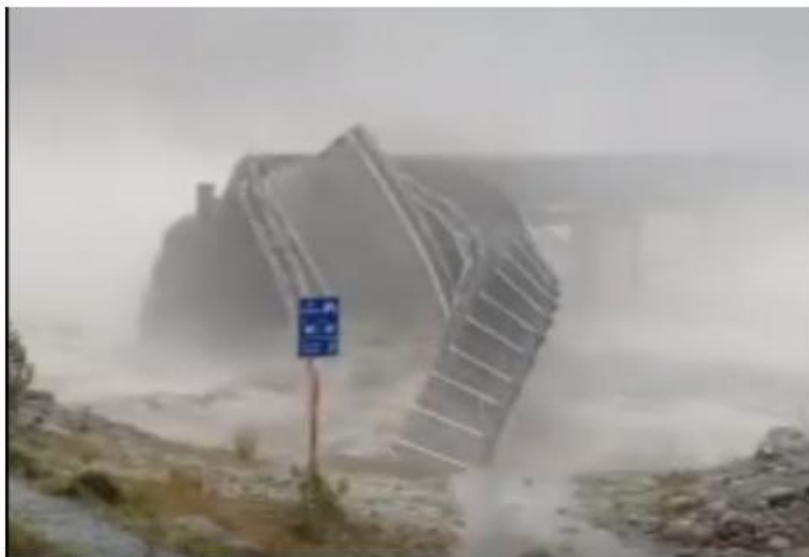
Motorway bridge over Waiho River in New Zealand destroyed by extreme flooding. via Video
