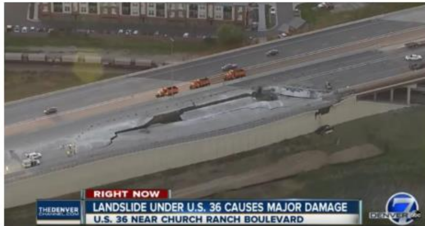
U.S. 36 highway collapsed between Boulder and Denver in Colorado. Picture via Youtube video
