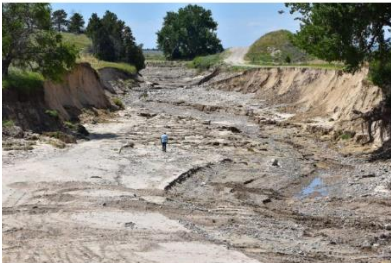
Irrigation tunnel collapses and cuts off 100,000 acres of farmland in Wyoming and Nebraska – Major threat for economy in both states. Picture: OFFICE OF WYOMING GOV. MARK GORDON
