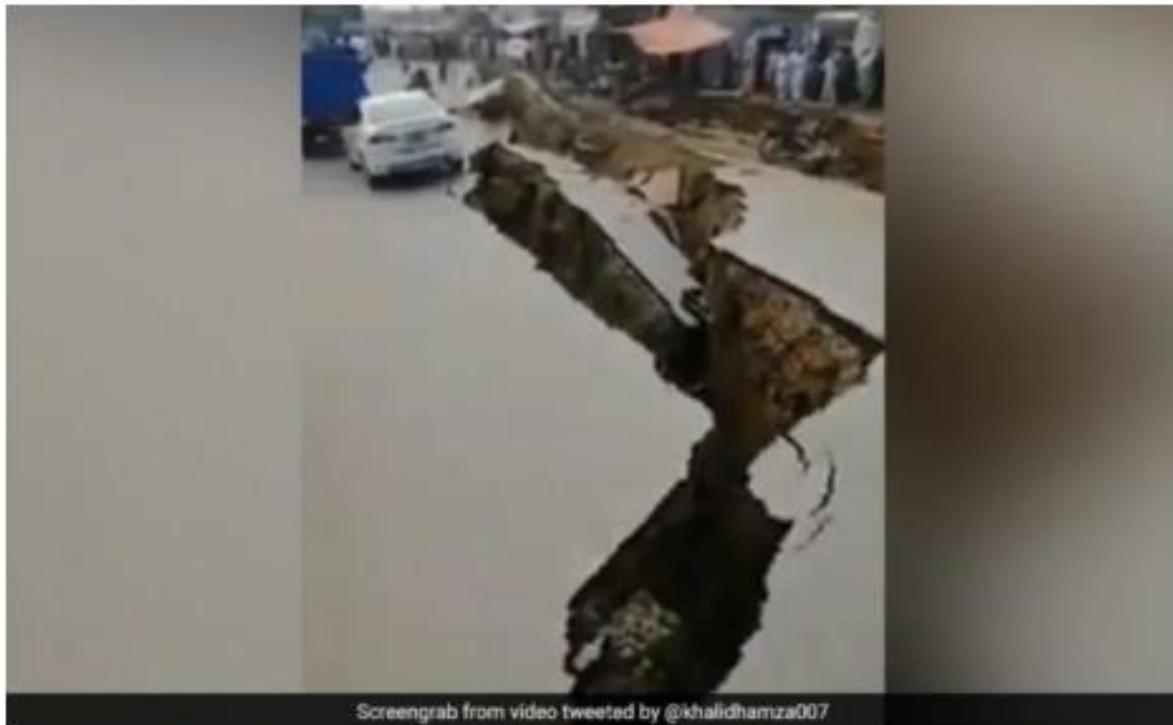
A deadly M5.8 earthquake hit Pakistan on September 24, 2019. Picture shows a crack in a road in Mirpur after the quake.
