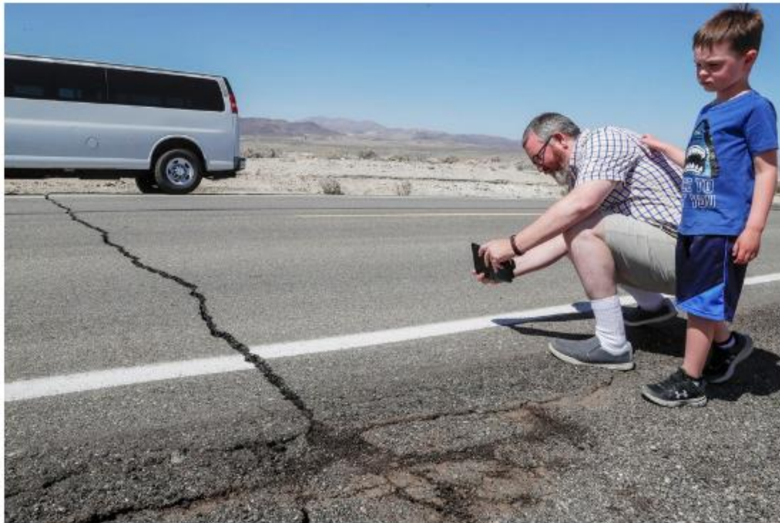
Andy Randolph and his son William stop for photos of a crack in California State Route 178 hours after a 6.4 magnitude earthquake struck the Searles Valley area on July 4, 2019 in Ridgecrest, Calif. ROBERT GAUTHIER, LOS ANGELES TIMES/TNS
