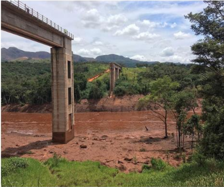
Iron ore railway bridge destroyed by mudflow, 3 kilometres (1.9 mi) downstream from collapsed dam killing 259 last year, Wikipedia
