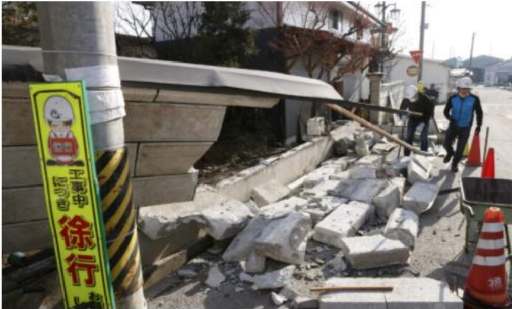
A collapsed wall by a strong earthquake is pictured in Kunimi, Fukushima Prefecture, Japan on Feb. 14, 2021. (Kyodo/via Reuters)
