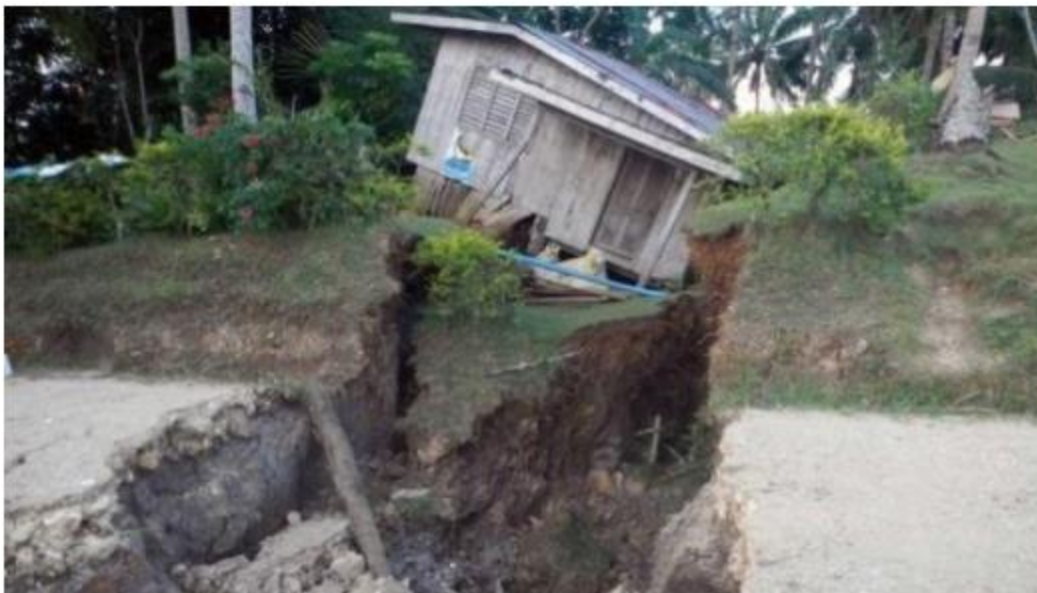
A house almost swallowed up by one of the cracks in the ground of the Philippines. Picture via Facebook
