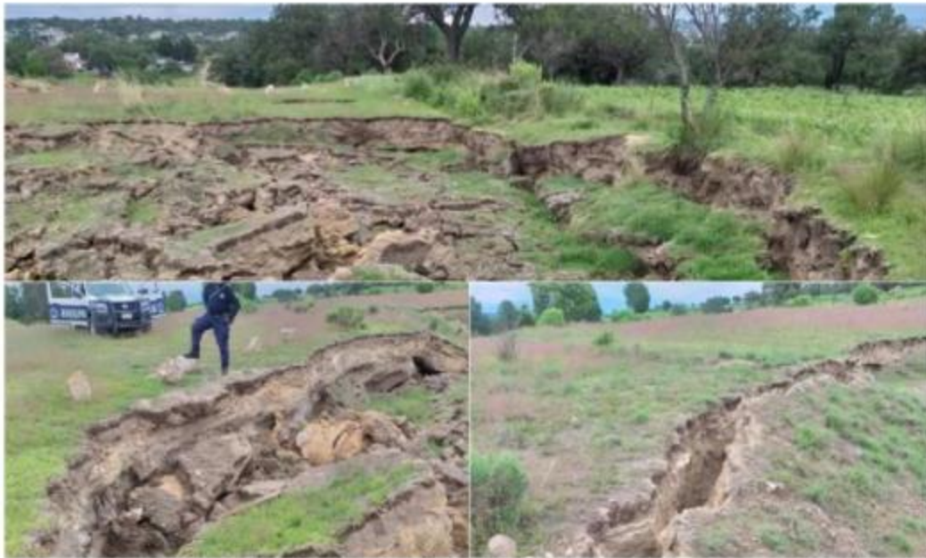
Is another giant sinkhole forming in rural Mexico? Huge cracks open up in Xaloztoc, Tlaxcala. Picture: El Pintero
