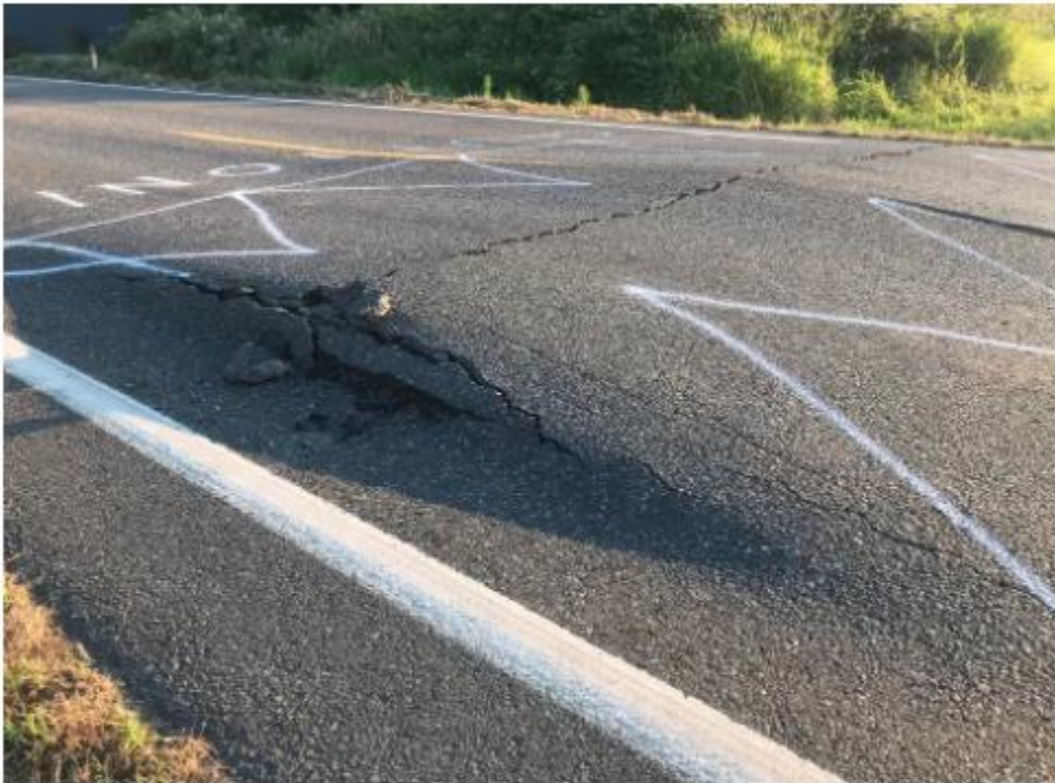
Transport infrastructure, such as roads and trains, have been drastically impacted by the heatwave hitting the area. Experts believe this is what is expected due to the climate crisis. (National Weather Service)
