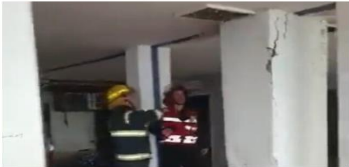
Cracks that appeared in a building in Tiberias following an earthquake on January 23, 2022, prompting an evacuation of residents. (Screenshot: Twitter)
