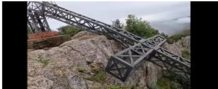
Cross vandalism in France
