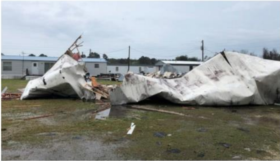
Tornado damage in Alabama. Picture via Brendan Kirby
